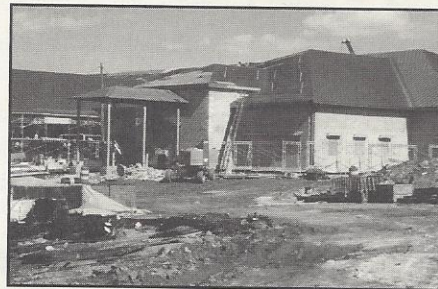
Construction days on new site
